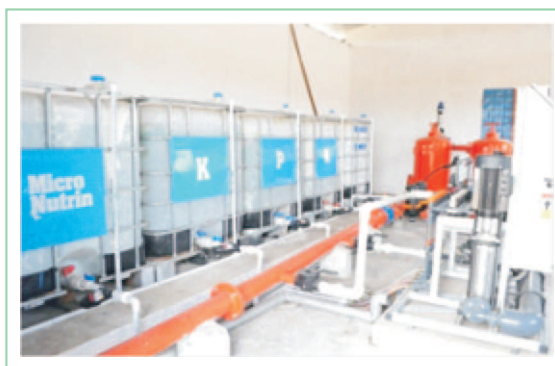
Fertigation unit (Netaject) installed at NRCP during 2013-14 for improving water and nutrient use efficacy
