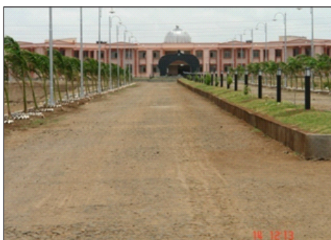
Fig.5: Newly constructed office-cum-laboratory of NRCP at Kegaon
